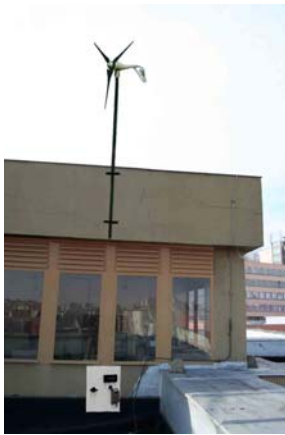
Figure 2 The turbine installation
