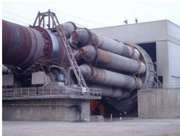
Figure 7 The cement kiln
