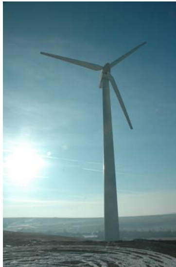
Figure 16 'Bükkaranyos' V-27 wind turbine
