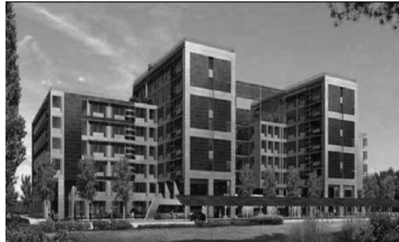
Fig.6 The Green Office in Meudon
