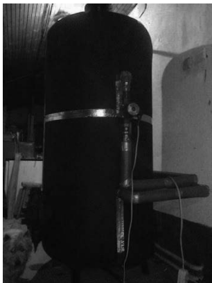
Picture 3. Storage tank during installation
