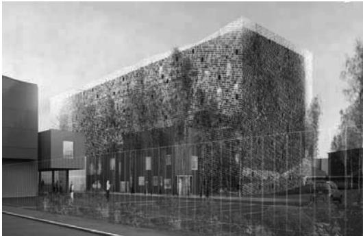
Fig.7 An archives building
