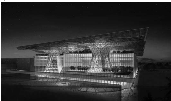
FIG.8 MASDAR HEADQUARTERS, ABU DHABI
