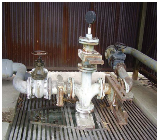
Fig. 1 Head of geothermal well FGT-1
