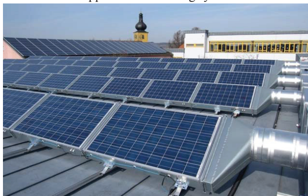
Figure 11. PVT hybrid collectors installed on the roof of a German swimming pool [27]
