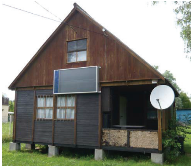
Figure 8. Hungarian summer cottage with solar air heater on its facade
