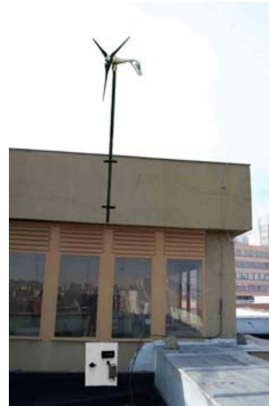
Figure 2.2.2 The turbine installation
