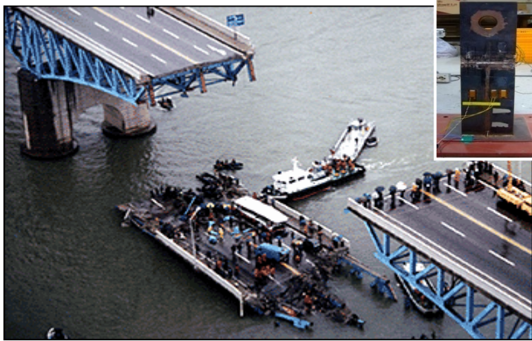
Sungsoo Bridge, Seoul (1994)
