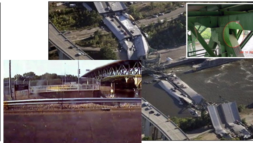
Highway Bridge, Minnesota (2007)
