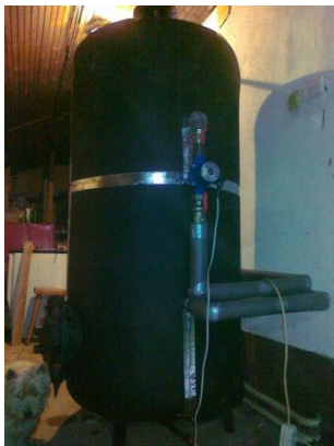
Picture 3. Storage tank during installation
